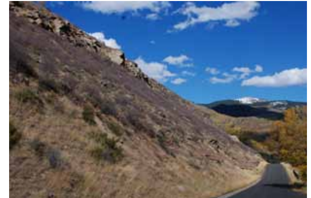
Rockfall and steep slope hazards in the Lionsridge neighborhood.
