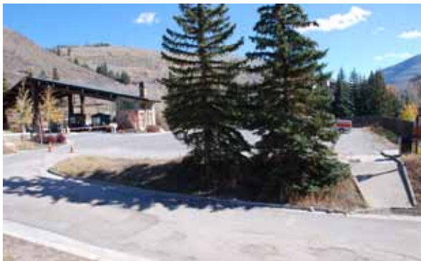
Development at the East end of Lionshead Parking Structure has been studied in the past.
